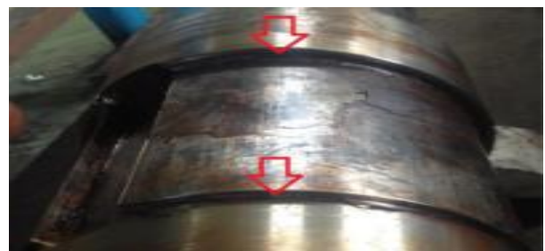
Fig. 38 Cracks at stress concentration points of the diameter change location
